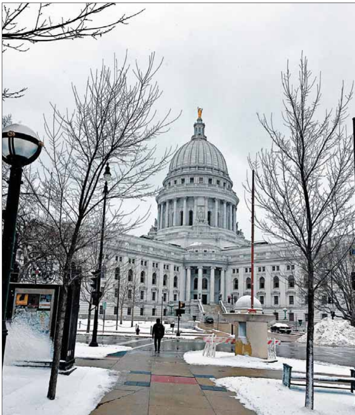
Wisconsin's Capitol building was completed in 1917 and dominates the skyline in downtown Madison.
